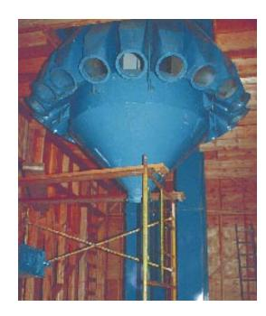
Above: A typical Roto-Flo during installation. Visible in the background are the leg sections of the Gerber Bucket Elevator; an excellent companion to the Gerber Roto-Flo. This installation required a special color to match existing equipment.
